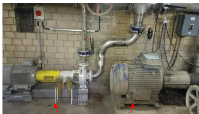
New pump – old pump
