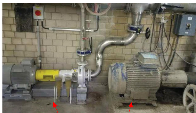
New pump – old pump
